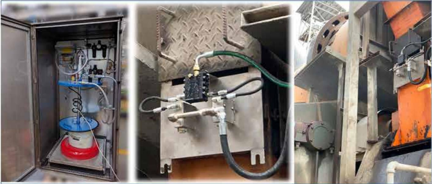
The use of lubrication systems is even more indispensable for the correct operation of machines when they operate in difficult environmental conditions such as those in cement and raw material processing plants. The installation of an automatic lubrication system allows machine down times to be reduced and allows consumption of the lubricant to be controlled and the life of the bearings, chains and gears to be increased.
