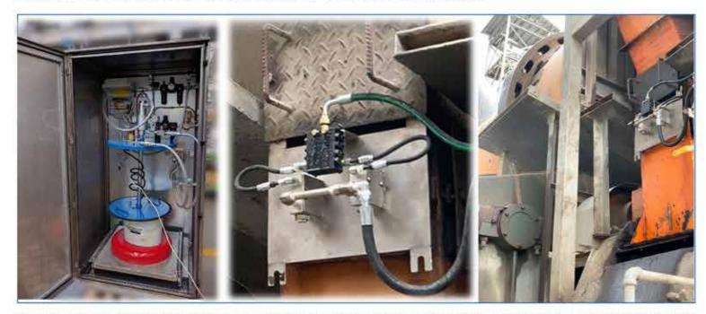
The use of lubrication systems is even more indispensable for the correct operation of machines when they operate in difficult environmental conditions such as those in cement and raw material processing plants. The installation of an automatic lubrication system allows machine down times to be reduced and allows consumption of the lubricant to be controlled and the life of the bearings, chains and gears to be increased.
