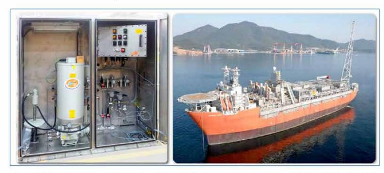
The use of lubrication systems is even more indispensable for the correct operation of machines when they operate in difficult environmental conditions, such as those in the Offshore. The installation of an automatic lubrication system allows machine down times to be reduced and allows consumption of the lubricant to be controlled and the life of the bearings, chains and gears to be increased.
